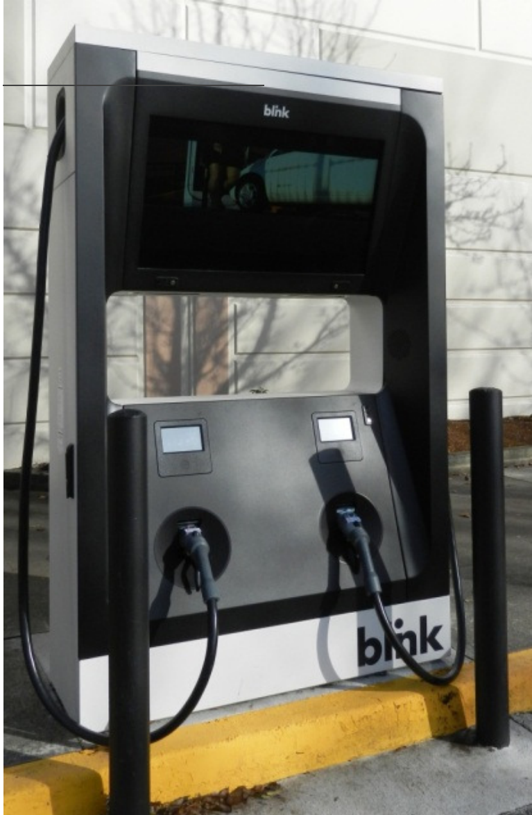
FIGURE 12: DC FAST CHARGER
